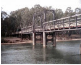
B6942 Cobram Bridge
