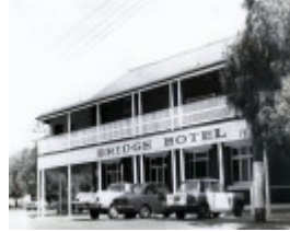
B2389 Bridge Hotel Nathalia
