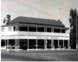
B2389 Bridge Hotel Nathalia
