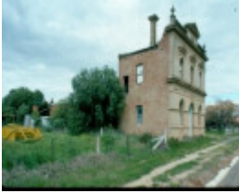
B4123 Former Mechanics' Institute
