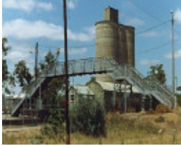
B5953 Goods Shed & Footbridge
