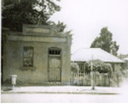
B3650 Blacksmith Shop & Cottage
