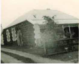
B4288 Former Bluestone Police Station
