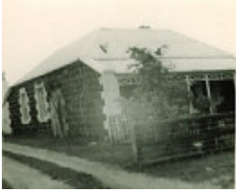
B4288 Former Bluestone Police Station
