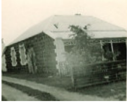
B4288 Former Bluestone Police Station
