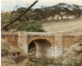
B1589 Djerriwarrh Creek Bridge
