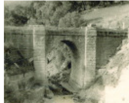
B1589 Djerriwarrh Creek Bridge
