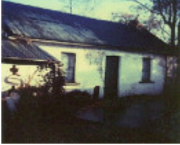
B5548 Ellerslie Cottage & Storeroom
