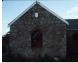
B2309 Stables end wall
