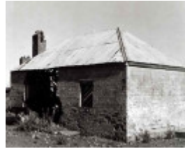
B2226 Glengower Homestead Cook House
