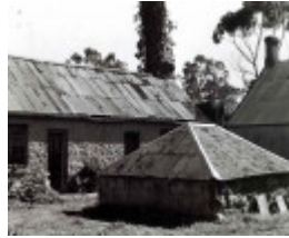
B2226 Glengower Homestead Underground Water Tank
