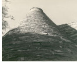
B1762 Ruins of Duke of Cornwall Mine
