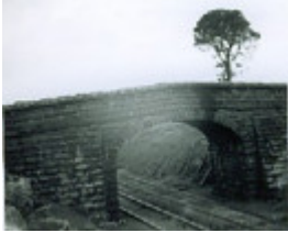
B2993 Humped Bridge Calder Hwy Taradale
