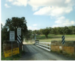
B6850 Zeal Bridge
