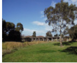
B6955 Winters Flat Bridge
