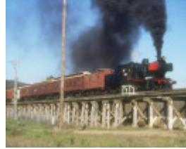
B6955 Winters Flat Bridge
