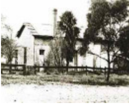
B1955 Former Castlemaine Courthouse
