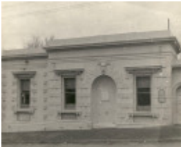
B0313 fmr State Savings Bank & Police Station Castlemaine
