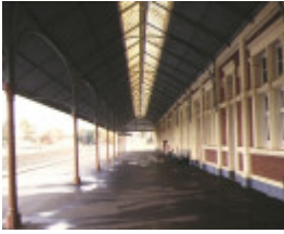
maryborough railway station platform view
