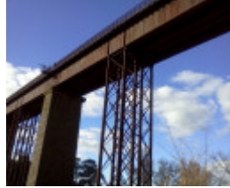
B1234 Taradale viaduct
