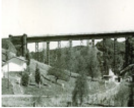
B1234 Railway Viaduct Taradale
