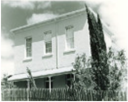
b3865 Aitken House 36 Johnstone St Castlemaine
