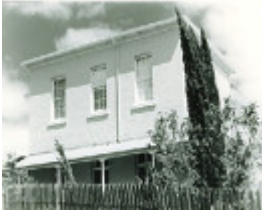
b3865 Aitken House 36 Johnstone St Castlemaine
