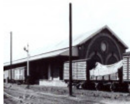
B3849 Castlemaine Railway Goods Shed
