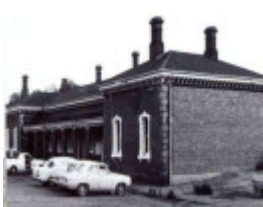
B3849 Castlemaine Station Entrance
