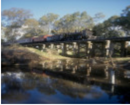
B6981 Muckleford Creek bridge
