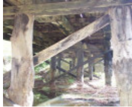
B7172 Todds Bridge piers
