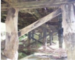
B7172 Todds Bridge abutment
