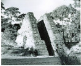
B1979 Garfield Water Wheel Base North St Chewton
