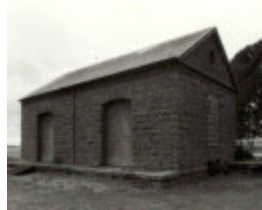
B3931 Bluestone Goods Shed
