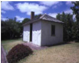
mccrae homestead charles street mccrae kitchen rebuilt
