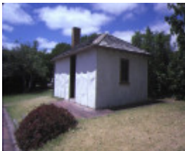
mccrae homestead charles street mccrae kitchen rebuilt
