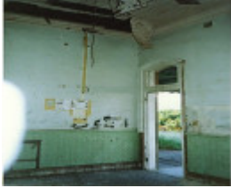
B5431 Railway Station, Koroit pre restoration
