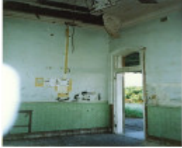
B5431 Railway Station, Koroit pre restoration
