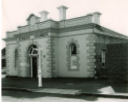
B0333 Former Post Office & Borough Chambers PORT FAIRY"
