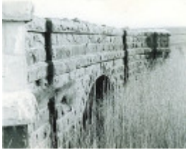
B0789 Burcharts Creek bridge
