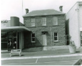
B2266 Cameron's Building, MORTLAKE
