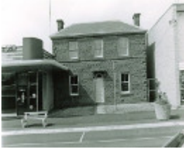
B2266 Cameron's Building, MORTLAKE
