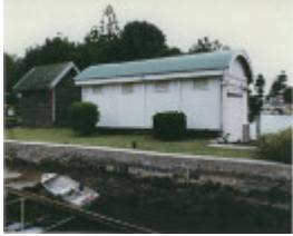
B5005 Former Boat Shed
