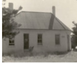
B0764 Former Merrijig Hotel
