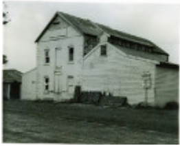
B0765 Warehouse/Butter Factory
