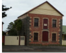
B0765 Warehouse/ Butter Factory
