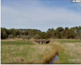
B7057 Burchett Creek Bridge (Google Earth image)
