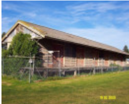
B7207 Railway Goods Shed
