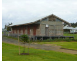
B7207 Railway Goods Shed
