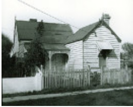
B1626 Mott's Cottage Sackville St Port Fairy
