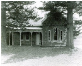
B4286 Frmr Shire Office Mortlake
