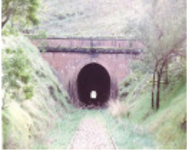
B5486 Cheviot Railway Tunnel
