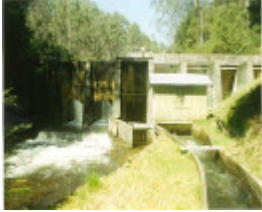
B6467 Rubicon Hydro Electric Power Scheme
