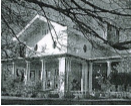
B1456 Alanvale Homestead, Campbells Bridge
