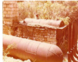
B4361 power plant, Heatherlie Quarry, Ledcourt
