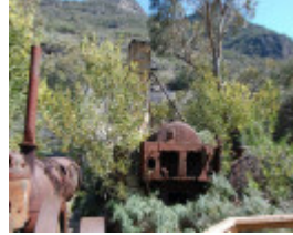
B4361 Heatherlie Quarry power plant
