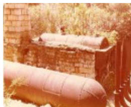
B4361 power plant, Heatherlie Quarry, Ledcourt
