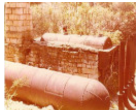
B4361 power plant, Heatherlie Quarry, Ledcourt
