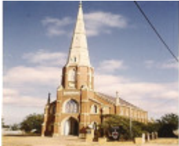
"B1699 St Matthews Uniting Church, Stawell"
