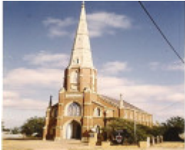
"B1699 St Matthews Uniting Church, Stawell"
