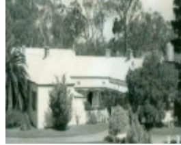
B1319 Tottington Homestead Courtyard
