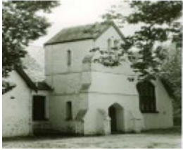
B1879 Anglican Parish Hall
