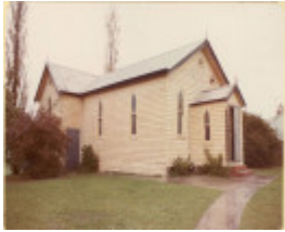
B5013 Former Methodist Church
