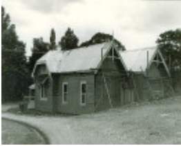
B4925 Former Post Office
