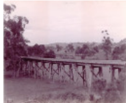
B6952 Tarwin River East Branch Railway Bridge
