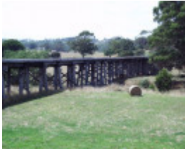
B6952 Tarwin River East Branch Railway Bridge
