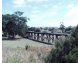
B6952 Tarwin River East Branch Railway Bridge
