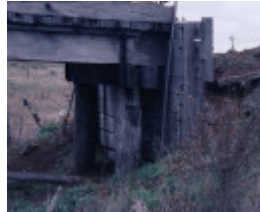
B6909 Railway Bridge
