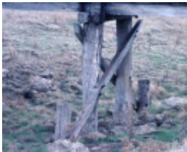
B6909 Railway Bridge
