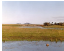
B6909 Railway Bridge
