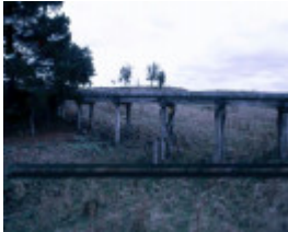
B6909 Railway Bridge
