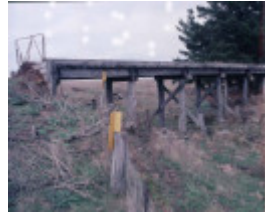
B6909 Railway Bridge
