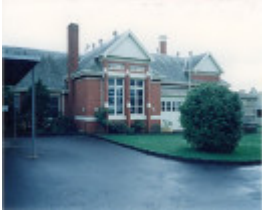
B6399 Hamilton Base Hospital Complex
