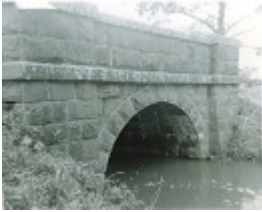
"B2817 Bluestone Bridge, Byaduk"
