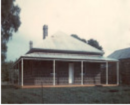
B3698 Lyne Homestead & Out Buildings
